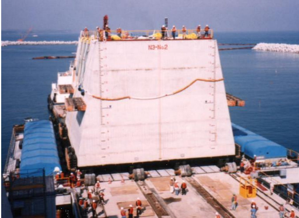
Figure G-11: Syncrolift Launching Concrete Caisson (Photo courtesy of RRNMI)
