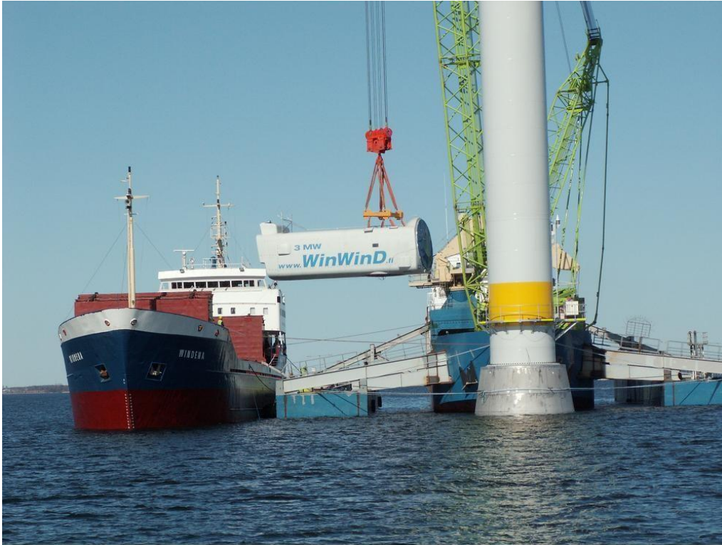
Figure 2-6: Lake Vänern Wind Turbines Installation
