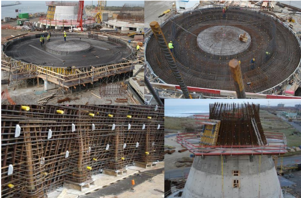
Figure G-10: Gravity Foundation Production Facility
