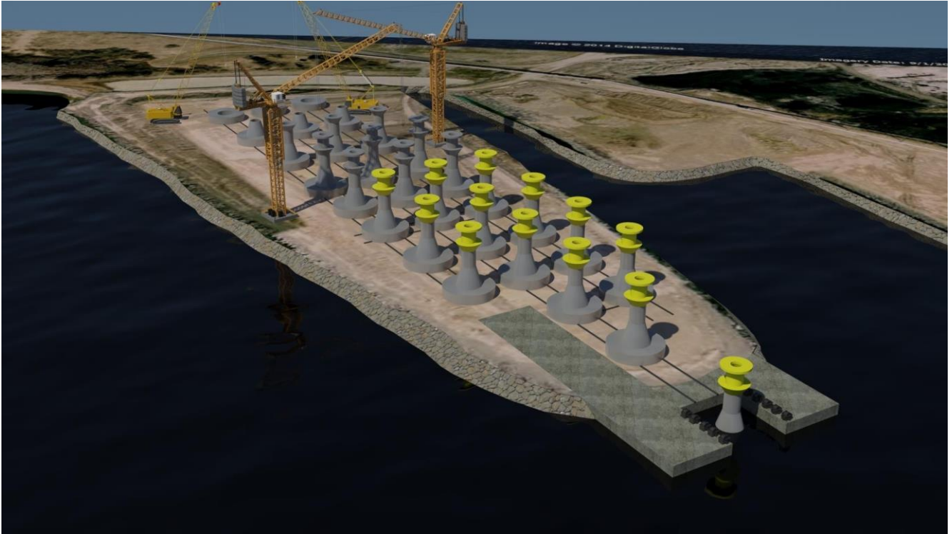
Figure G-13: Fabrication Facility with Foundation in Launch Position
