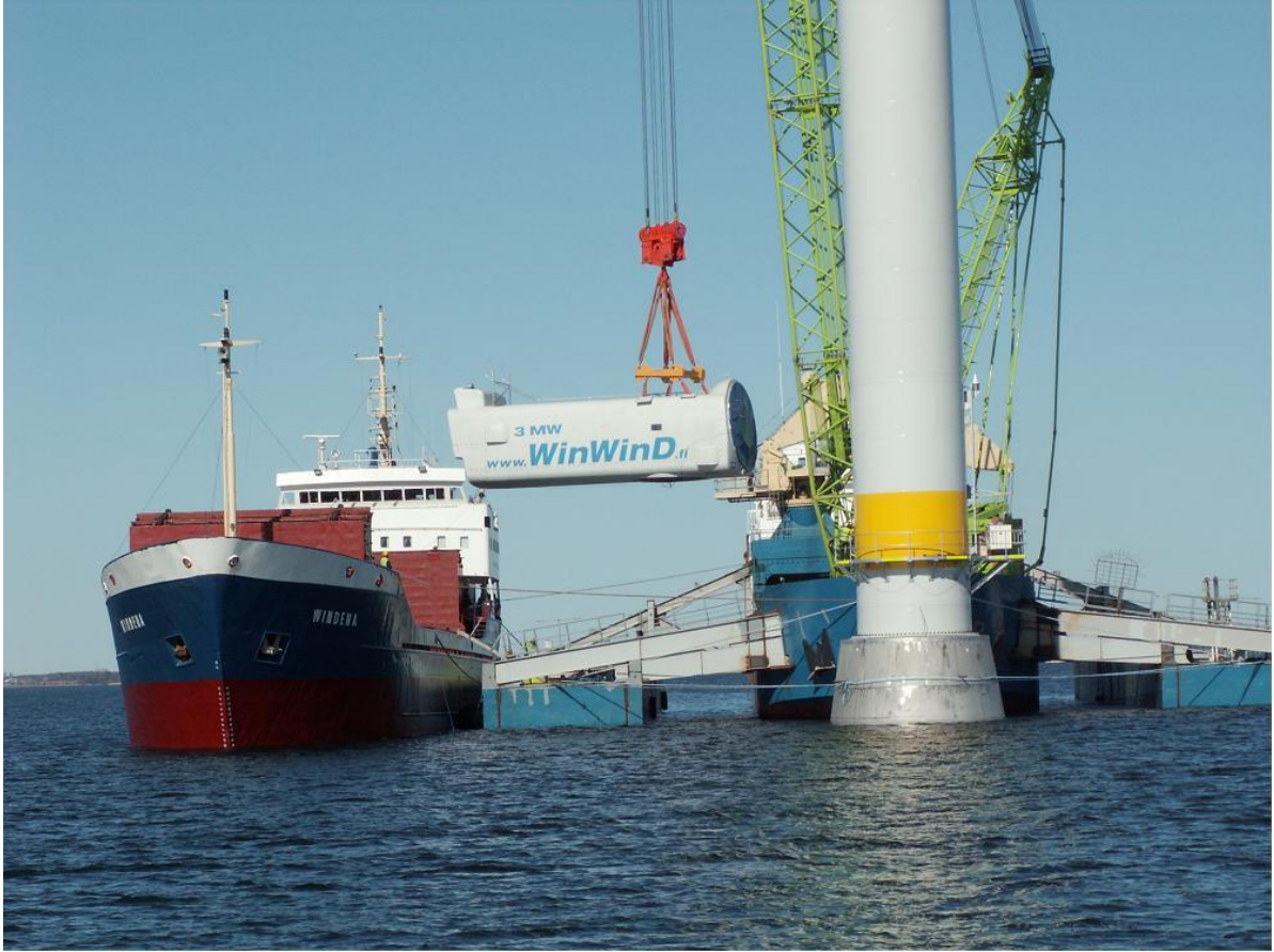
Figure 1-6: Custom WTG Installation Vessel at Lake Vänern
