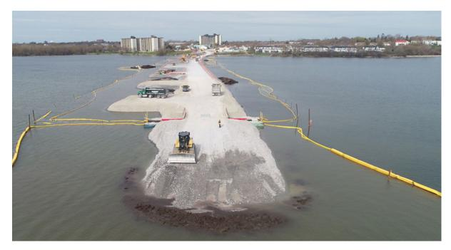
Figure A.71 - Third Crossing Construction Using a Temporary Causeway Across the Cataraqui River, Involves Dumping Fill Material in Provincially Significant Wetland,
